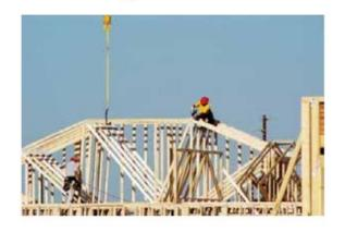
Engineered wood roof trusses provide a wealth of benefits for designers, engineers and construction professionals. The uniformity of their design make it easier to build pitch-perfect roofs. Designs can be more complex and trusses provide broader freedom with roofing styles for a greater aesthetic appeal. While they may cost a little more, they save on construction time and require less expertise to install.
